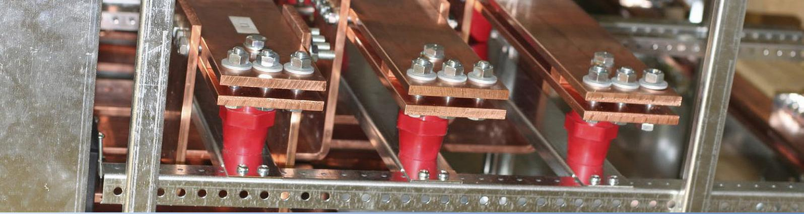
The temperature of electrical connections in power distribution systems is an important indicator of their condition. As connections degrade and fail, their resistance increases and their temperature can rise, causing further damage and a potential fire or explosion risk.
