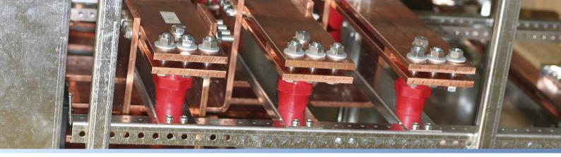
The temperature of electrical connections in power distribution systems is an important indicator of their condition. As connections degrade and fail, their resistance increases and their temperature can rise, causing further damage and a potential fire or explosion risk.
